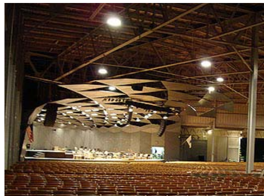
Figure 12: View of the canopy over the orchestra in the Tanglewood Music Shed. The canopy consists of open and closed sections of equilateral triangles of variable size. The canopy acts as a filter, directing high frequencies down into the orchestra and the first few rows of the audience, and letting the low frequencies into the upper reaches of the hall, where they have ample time to bounce around before coming
